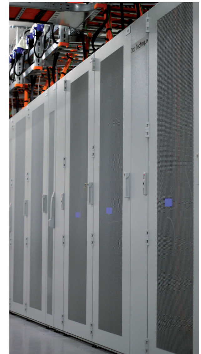
Racks 19" DK TS et LCP In Line de Rittal
